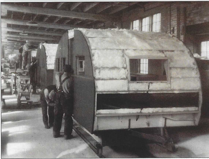
Above left: Men working on trailers at the Alma Trailer Company, c. 1938. Above right: A photo showing the cargo capacity of a trailer produced by Alma Trailer Company in 1938.
